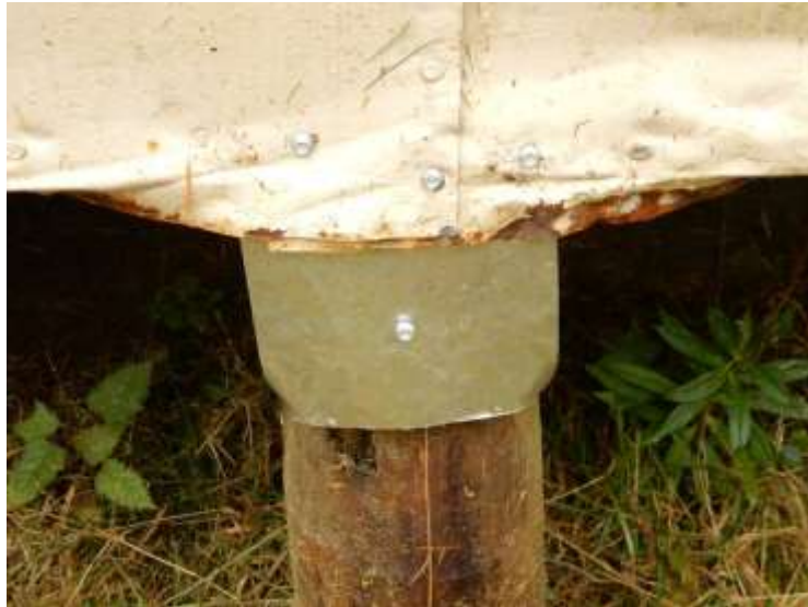
Above: Flashings on pile bearers
