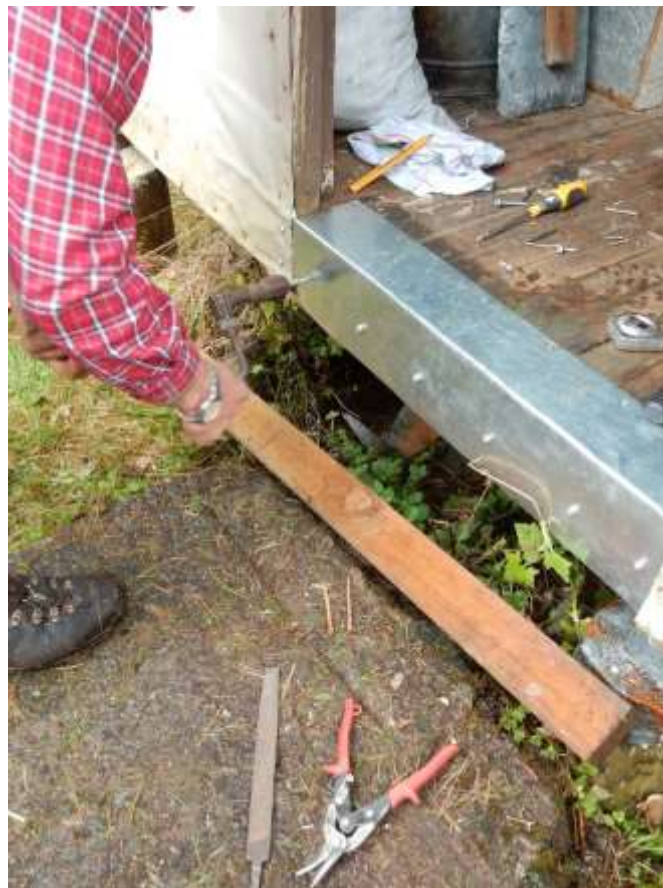
Above: Securing the new door sill flashing
