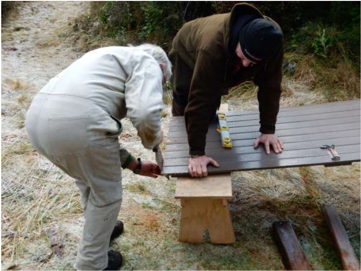
Above: Martin Clapham (L) & Craig Benbow (R) trimming the base of the door
