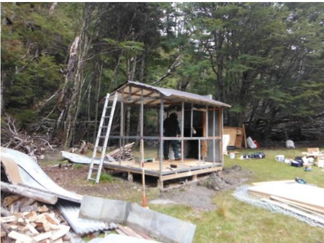
Ceiling on to provide bracing
