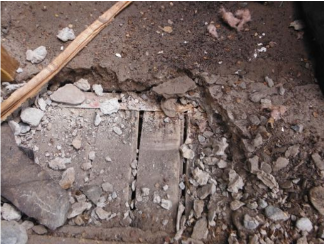
Floorboards under old hearth
