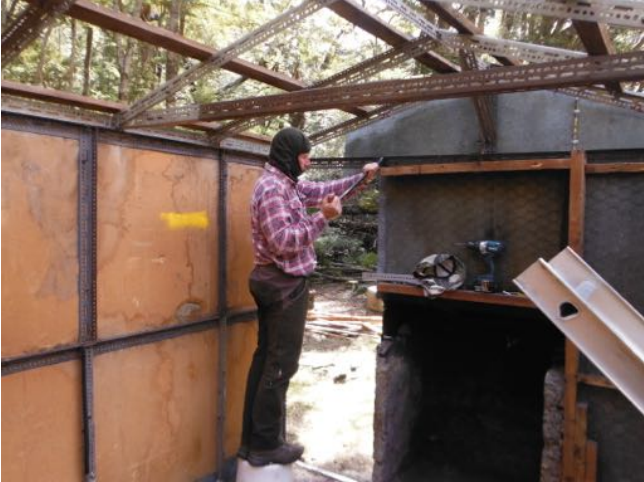
Ed stripping walls
