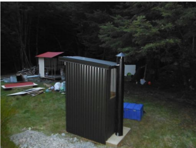
Toilet completed, hut roof on
