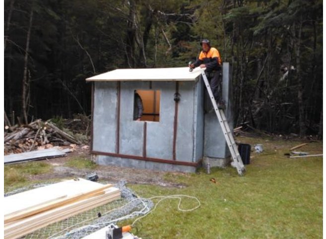
Mike fixing ply to roof
