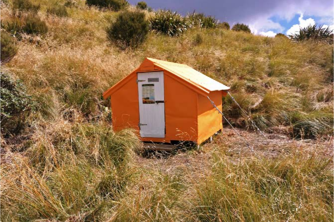
Newton Range Biv after work by Bruce McLelland and Permolat West Coast
