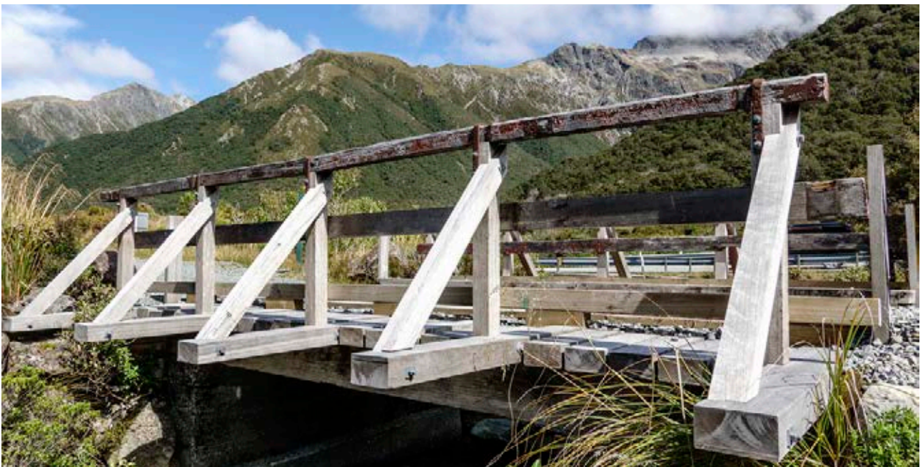
The restored Temple Basin Historic Bridge, Arthur's Pass National Park
