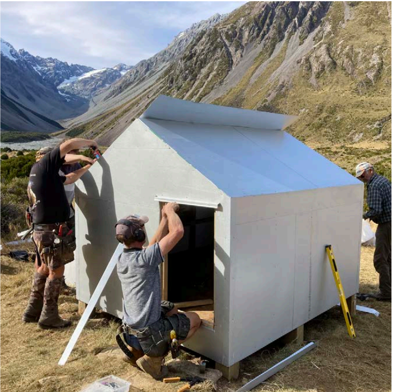
NZDA Ashburton renovating Lawrence Biv, Canterbury High Country
