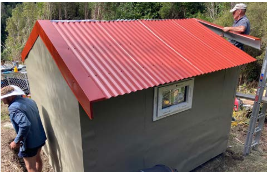
Renovating Rocky Creek Biv, West Coast
