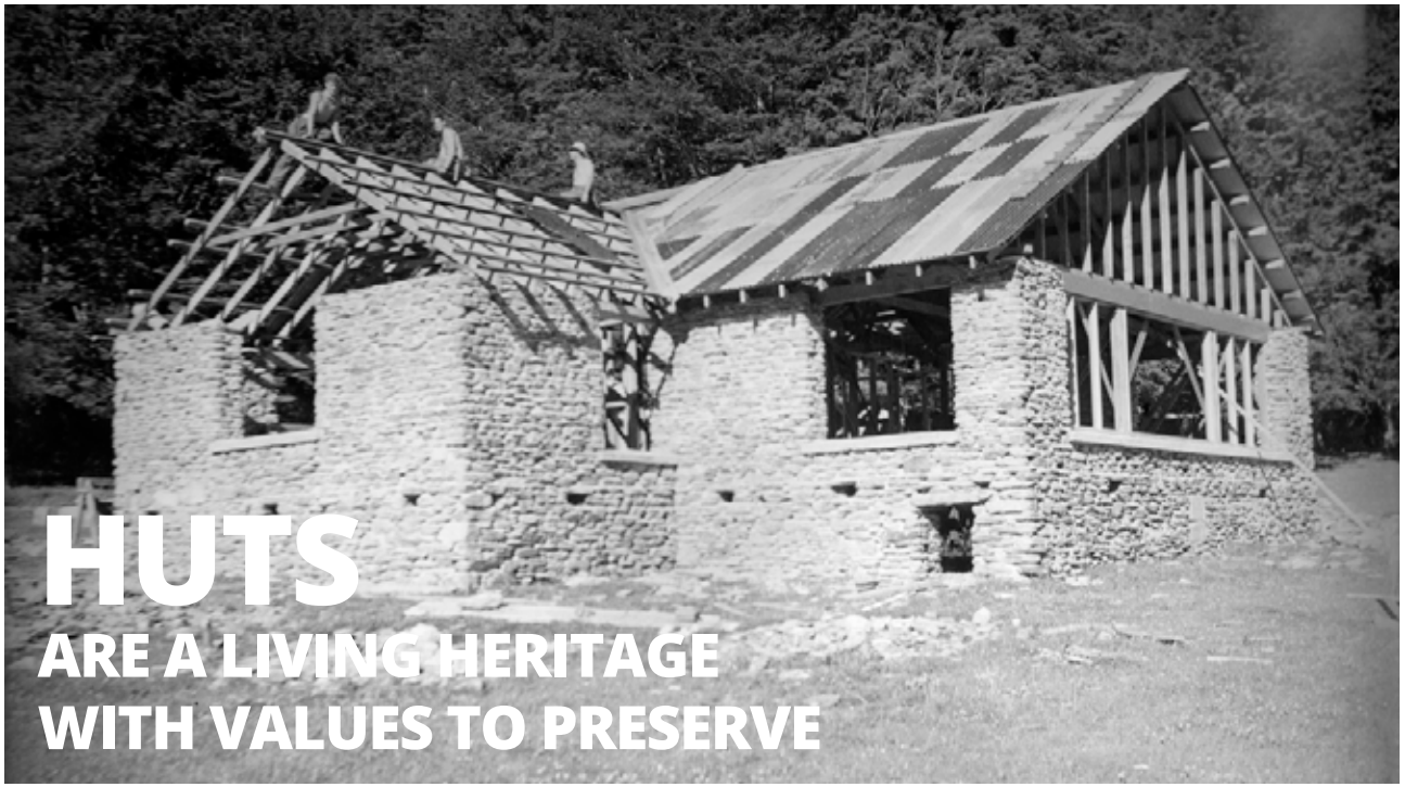
Aspiring Hut under construction, 1949
