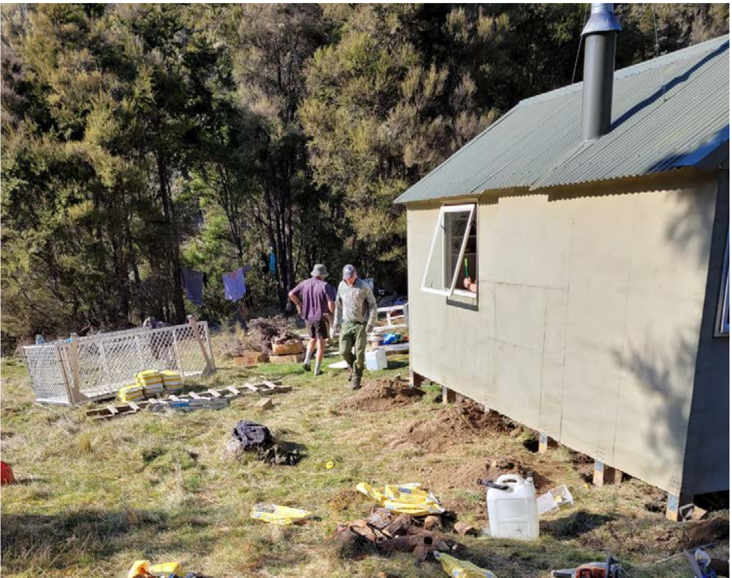
NZDA Marlborough and DOC re-piling Penk Hut, Ferny Gair Conservation Area
