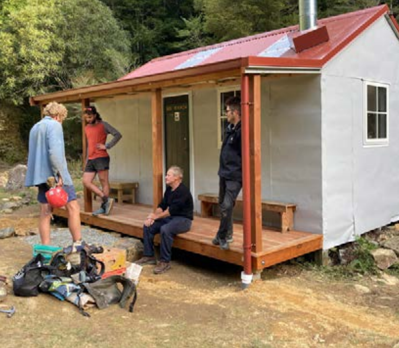
Mid Wairoa Hut renovation, Richmond Forest Park
