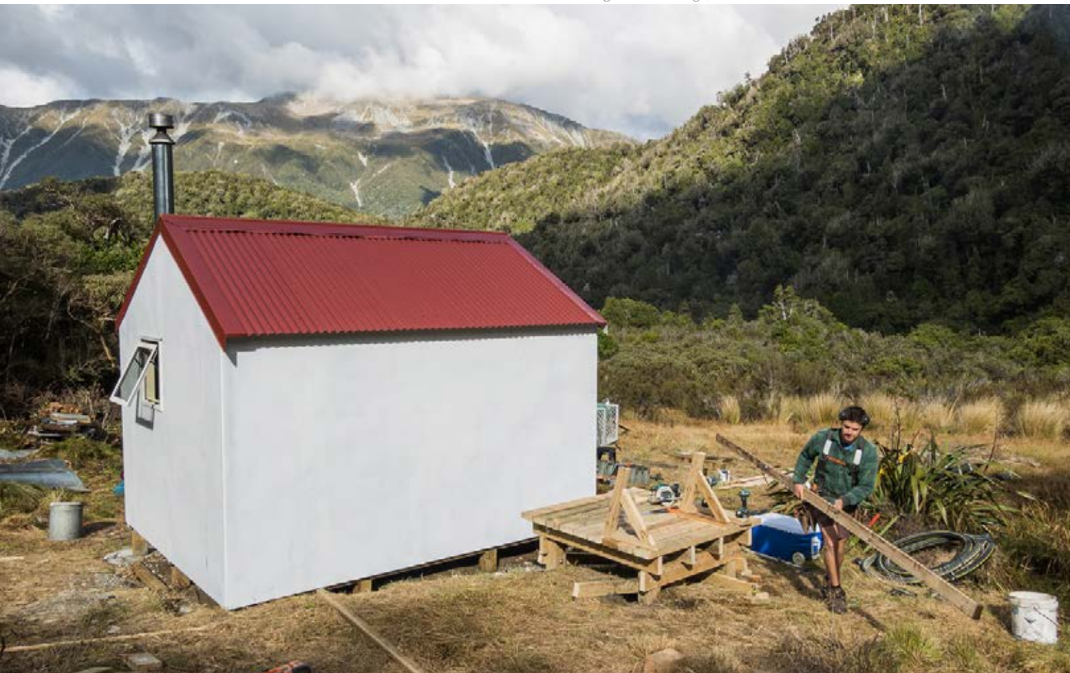
Lewis finishing Dunns Creek Hut rebuild.
