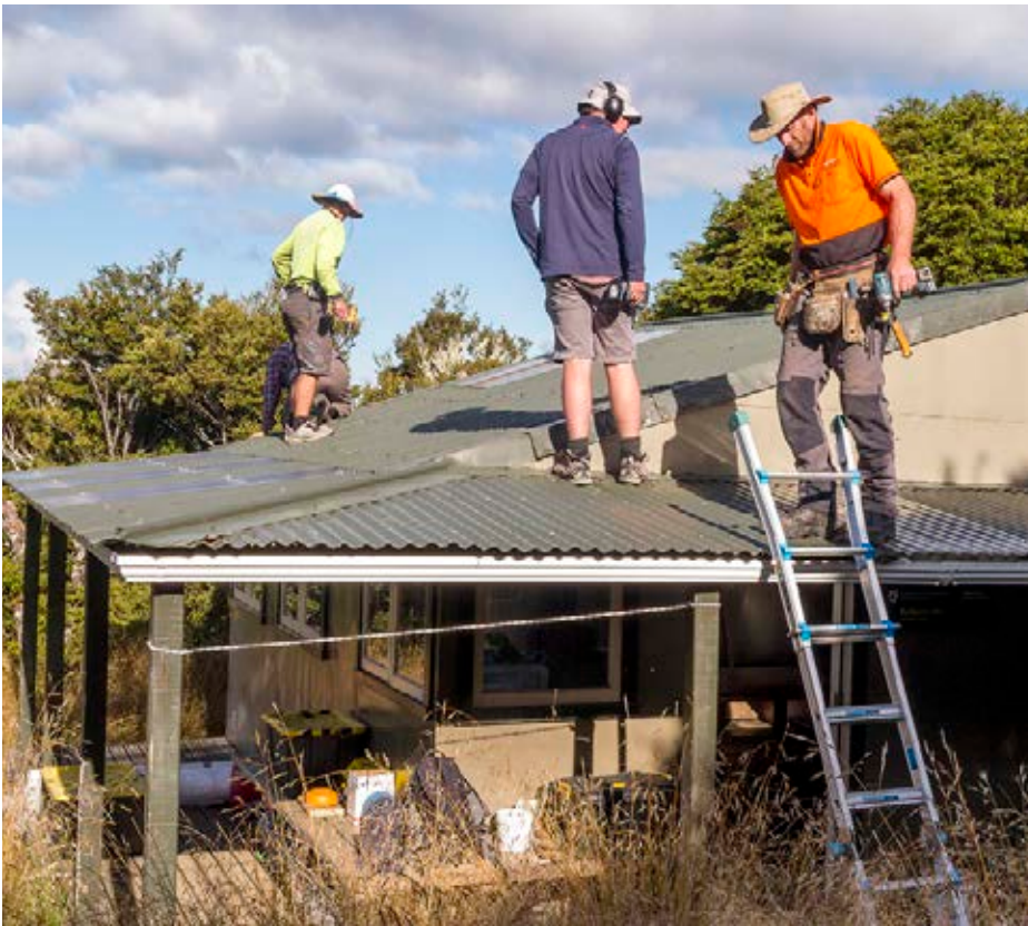
Re-roofing Balloon Hut, Kahurangi National Park
