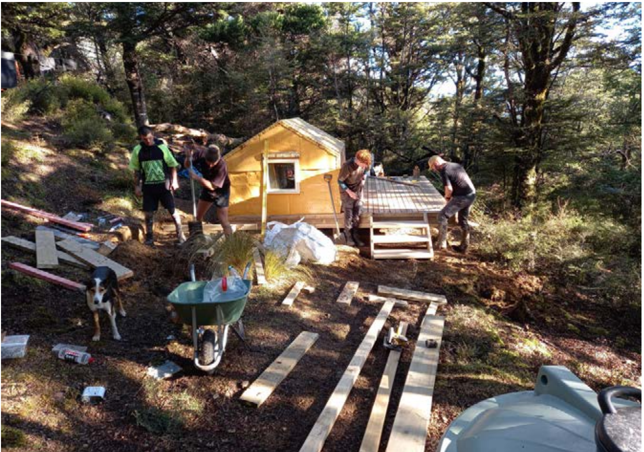
Fitting a deck and new water tank to Black Birch Biv, Kaweka Forest Park
