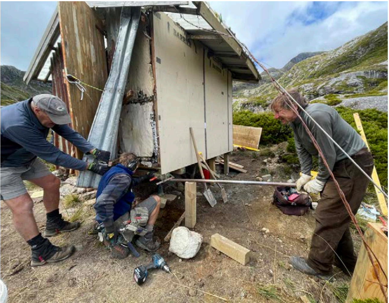
The NZAC team re-piling Robin Saddle Hut
