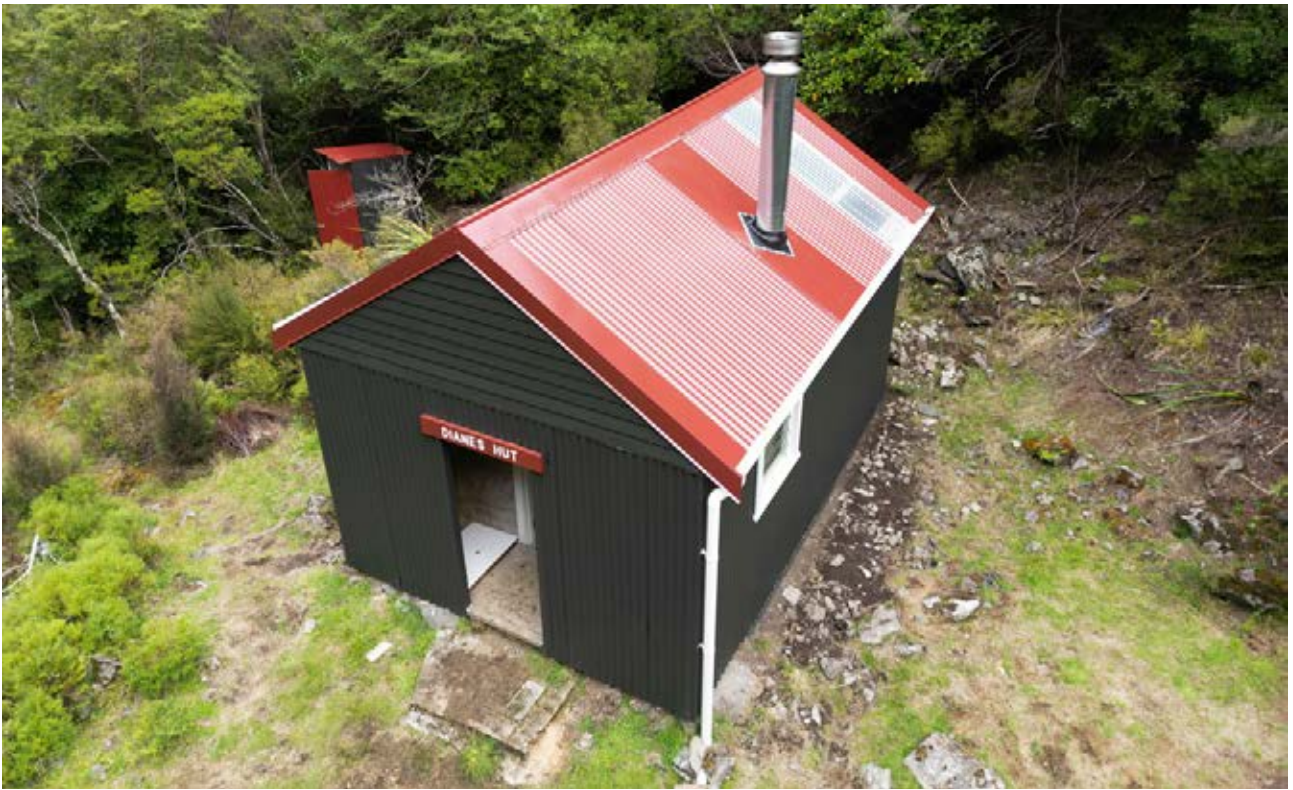
Diane's Hut after a full renovation, Ruahine Forest Park
