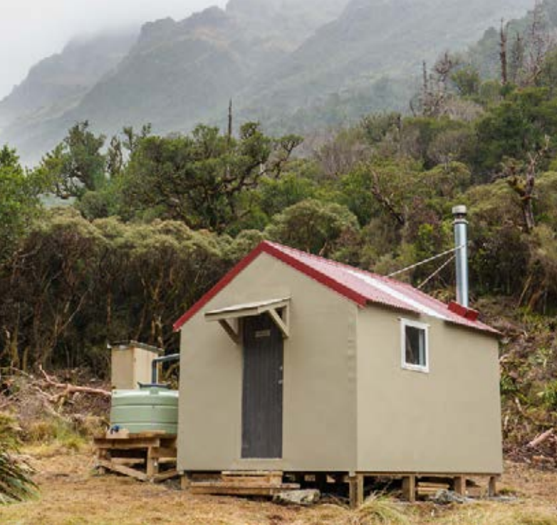
Dunns Creek Hut after restoration, West Coast
