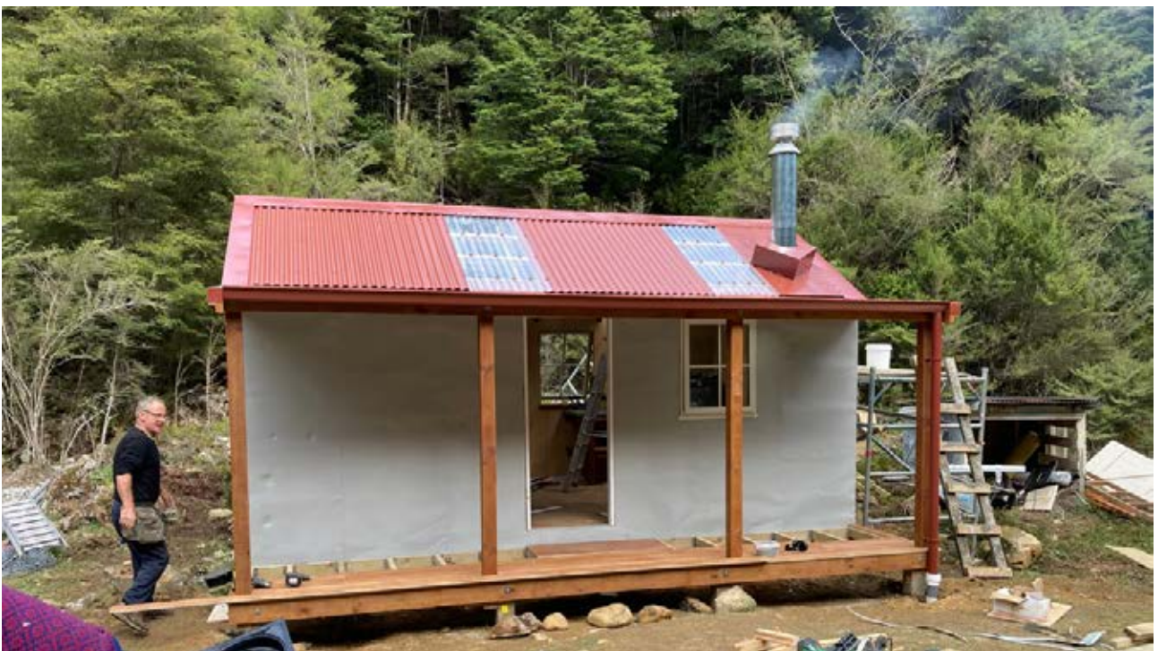
Finishing Mid Wairoa Hut renovation, Richmond Forest Park
