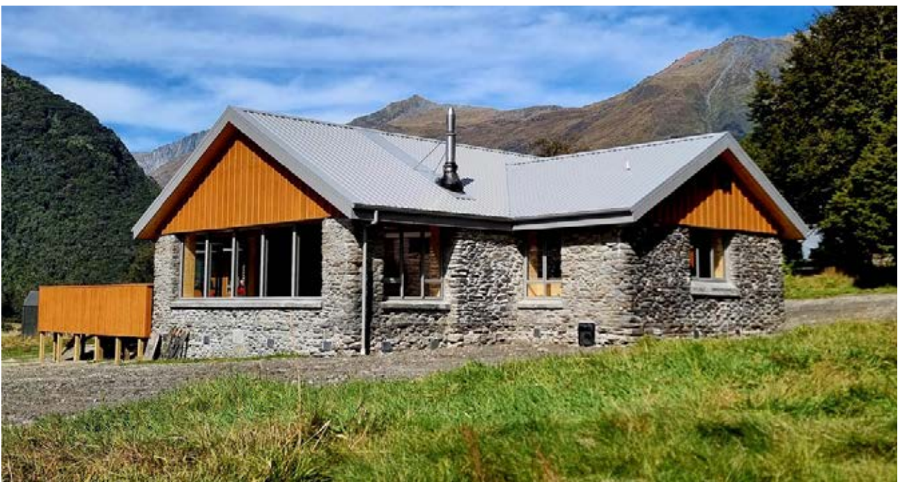
NZAC's Aspiring Hut after the 2022/23 rebuild
