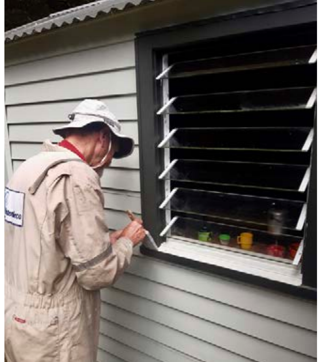
Painting Ellis Basin Hut, Kahurangi National Park
